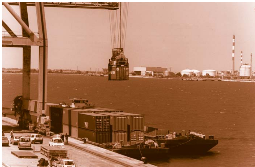
Port Autonome de Marseille - Communication/Service photo
